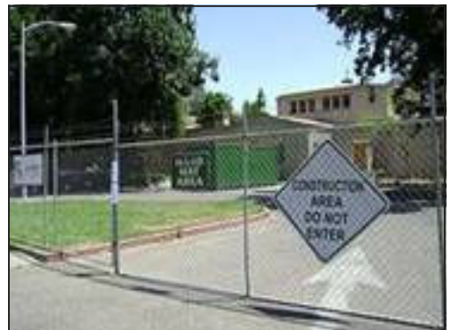
Visalia Library Branch Construction
