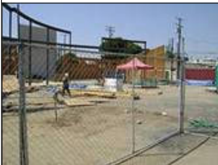
Lindsay Library Branch Construction
